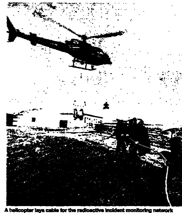
A helicopter lays cable for the radioactive incident monitoring network for which BT's Global Network Services will provide key elements
